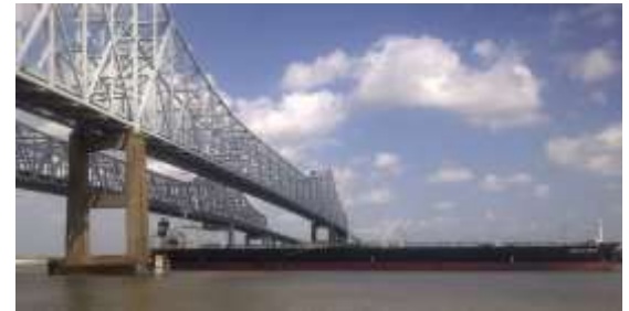
Figure 22. Tanker steaming northbound under the Crescent City Connection in New Orleans.
